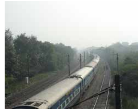
Railway Line near Ashram Chawk
