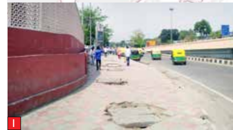
1 Unsafe footpaths with broken or missing manhole covers
