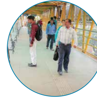
Grand Road Skywalk, Mumbai, India
