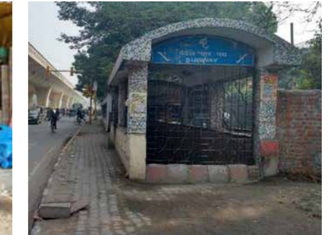
Low-maintained and poorly lit Subways
