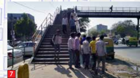
7 100% blockage by existing foot over bridge
