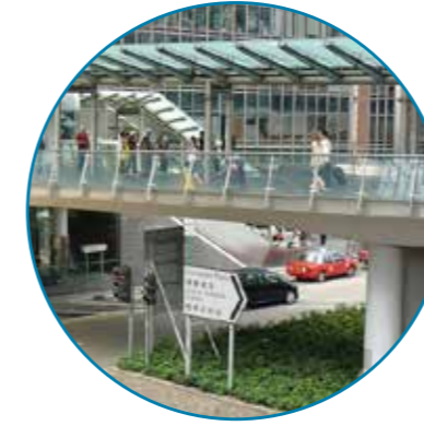
Connaught Road Skywalk, Central , Hong Kong, China
